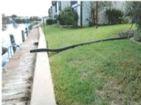
Picture 36 - Soils Eroding Away from Structures
