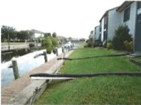
Picture 35 - Soils Eroding Away from Structures
